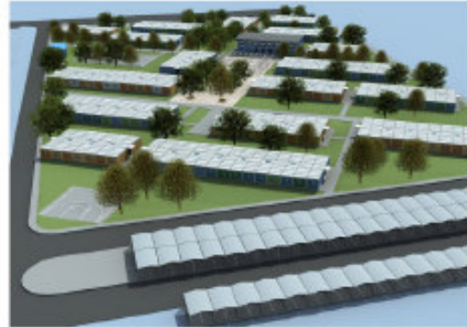
A working zone – recycling plant is a part of new Roma settlement
